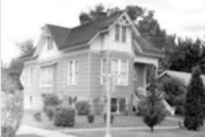
Salem House, Highland District, 1948.
