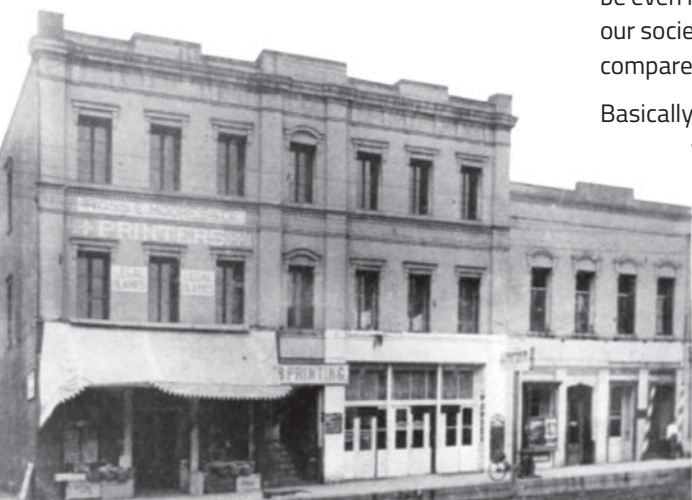
The Holman Building, on the NW corner of Commercial and Ferry streets in Salem, the location of our first meeting. The photo is from 1925.
